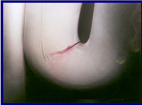
Close-up of crack
